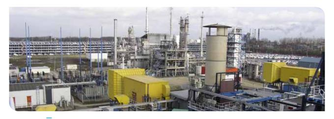
A CO-generator consists of a desalination plant and a boiler. Smallest organic impurities result in production of carbonic acid, which increases the risk of corrosion considerably. It is important to detect impurities quickly and reliably.
